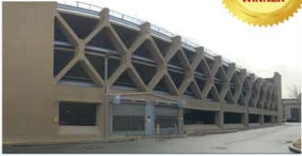
University of Pennsylvania, Walnut 32 Parking Garage
